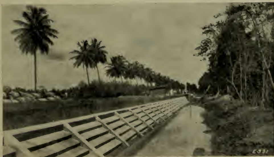
FIG. 8. REINFORCED CONCRETE FACED DAM. (10 STEPS.)
